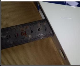
24. Measure the same length on the surface of the vertical and mark it out as picture.
